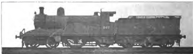
Fig. 5041. Eight-Wheel, Single Driver Locomotive. Great Northern Railway. Cylinders 19 in. x 26 in.; Working Steam Pressure 175 lbs. per sq. in.; Total Heating Surface 1,296.6 sq. ft.; Diameter of Drivers 92 in.; Weight on Drivers 49,760 lbs.; Total Weight 108,890 lbs.
